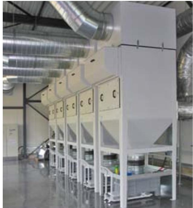
*ASD extraction and filtration technology can be a centralised solution for complete manufacturing halls.*
