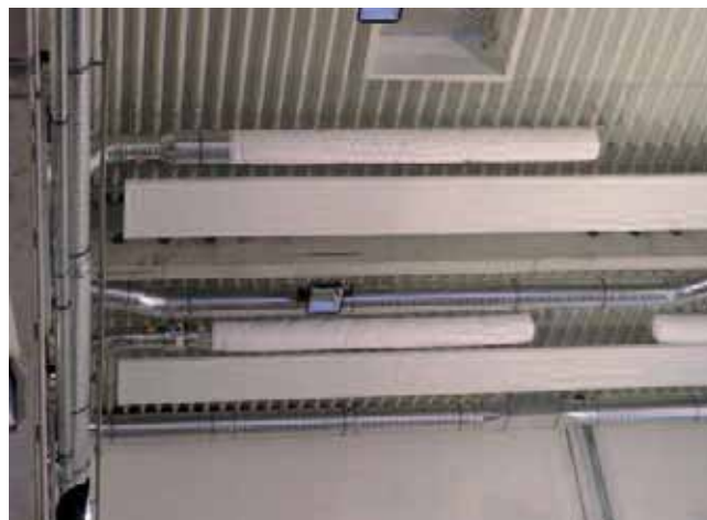
Fig. 2. Air supply under the ceiling
